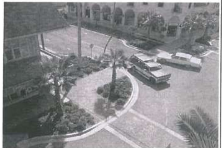
This bump-out reduced turning speeds by 6-8 MPH and reduced the pedestrian crossing distance and time exposed to traffic
